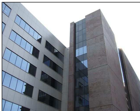
Fig. 1 Centraplaza in Canberra, Australia
