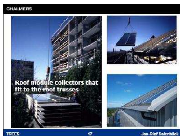
Solar collectors avoiding to repair a terrace roof
