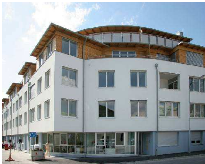
Fig. 4 Residential building “Pfarrhofgasse”
