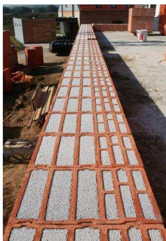
**Fig. 5** Masonry with clay block „Poroton T 8“
