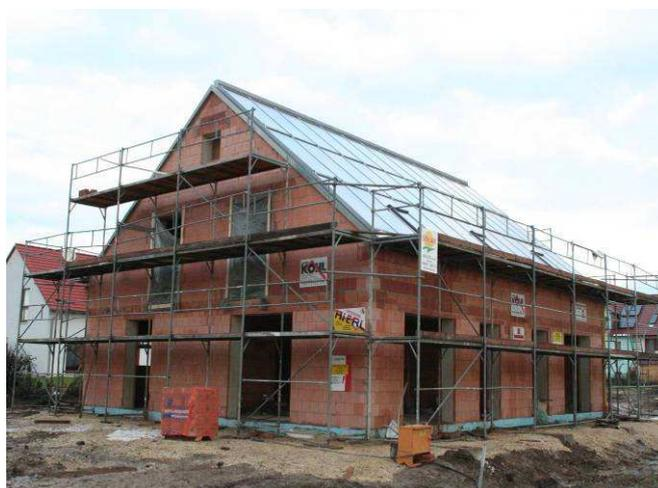
**Fig. 6** Outer wall with clay blocks „Poroton T 8“
