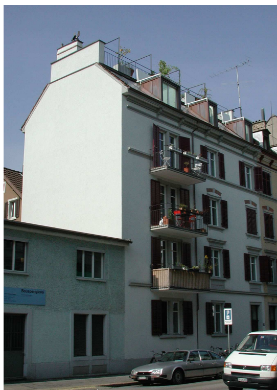
Fig. 1 Magnusstrasse 23, view from the street after renovation
