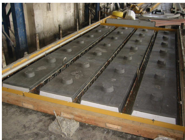
Fig. 5 Precast filigran panel with installation shell elements – during experimental manufacturing
