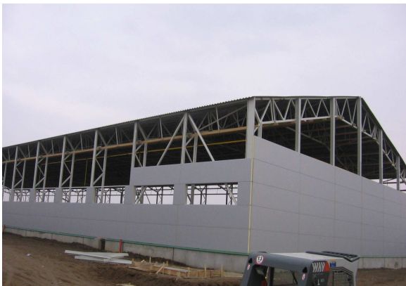
Fig. 3 Quick construction, rapid production
