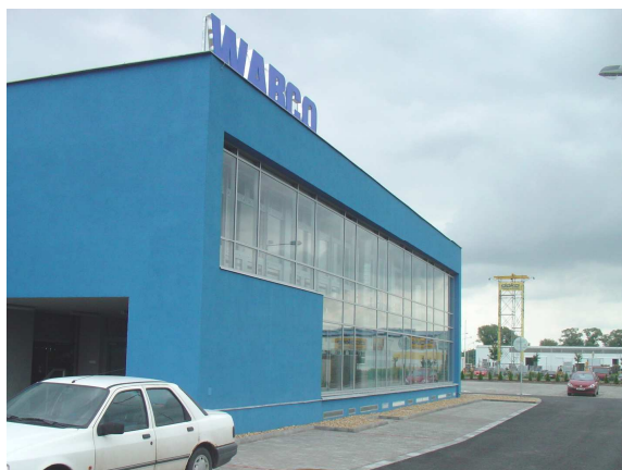
Fig. 1 Small double-skin solar energy façade
