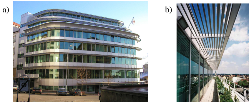
Fig. 3 Passive glazed façade of administrative building in Brno a) the south-west elevation b) local view of the façade with the sunscreen.
