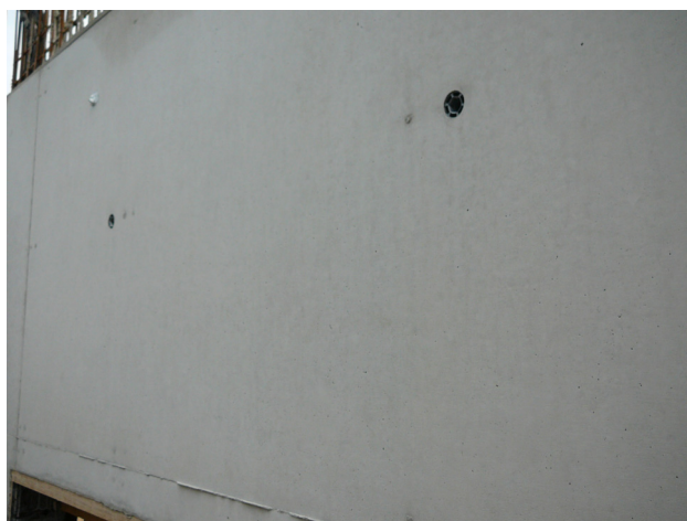
Fig. 5 View of finished wall
