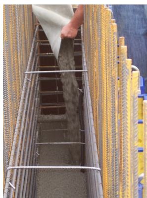
Fig. 2 Placing fresh concrete into formwork
